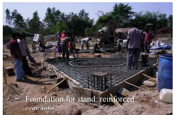
Foundation for stand: reinforced concrete
