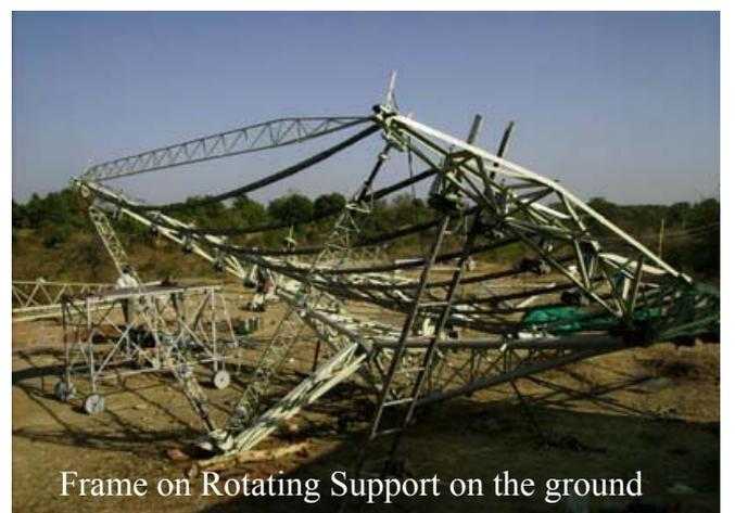
Frame on Rotating Support on the ground
